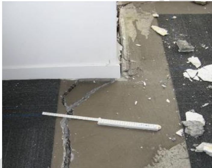
Figure C5.40: Observed separation between floor and supporting beam due to beam elongation in 2011 Canterbury earthquakes (Bull)
