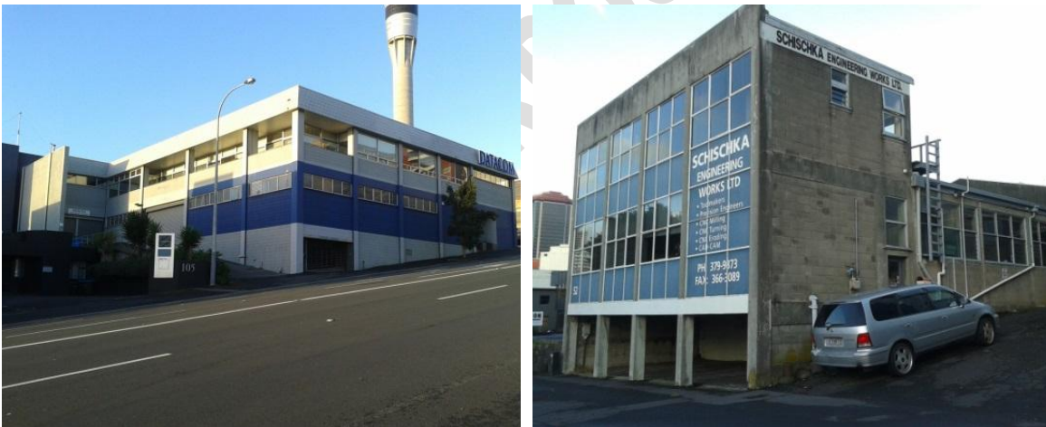
Figure C7.4: Examples of reinforced concrete frames with concrete block masonry infill (Laura Putri)
