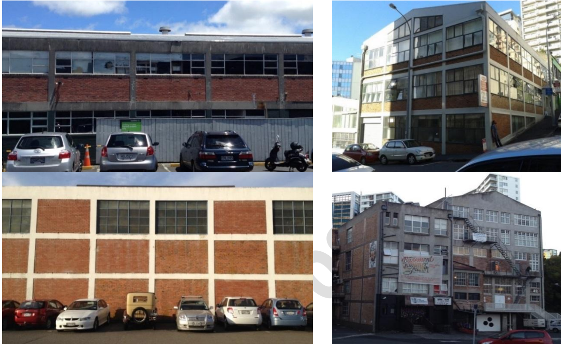
Figure C7.1: Examples of reinforced concrete frames with clay brick masonry infill (Kevin Walsh and Laura Putri)
