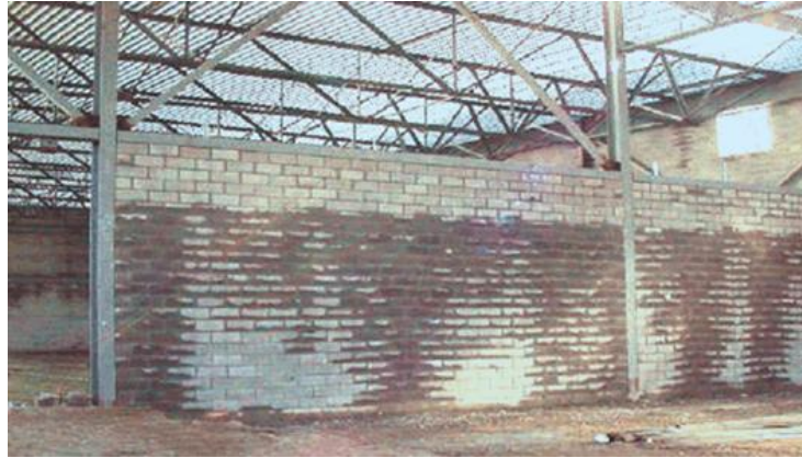
Figure C7.5: Examples of steel frame industrial building with concrete block infill (David Biggs)
