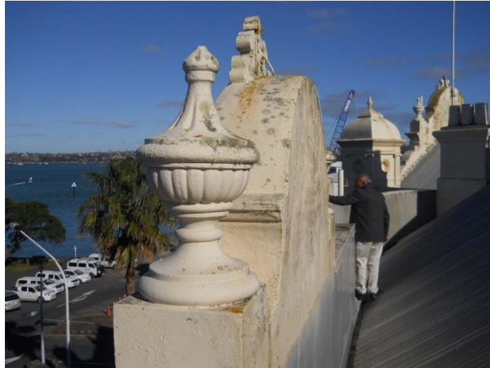
Figure 10.22: Secondary elements (Miyamoto International)
