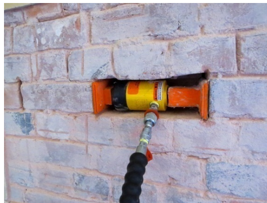
(b) In situ shear test without flat jacks (EQ STRUC Ltd)
