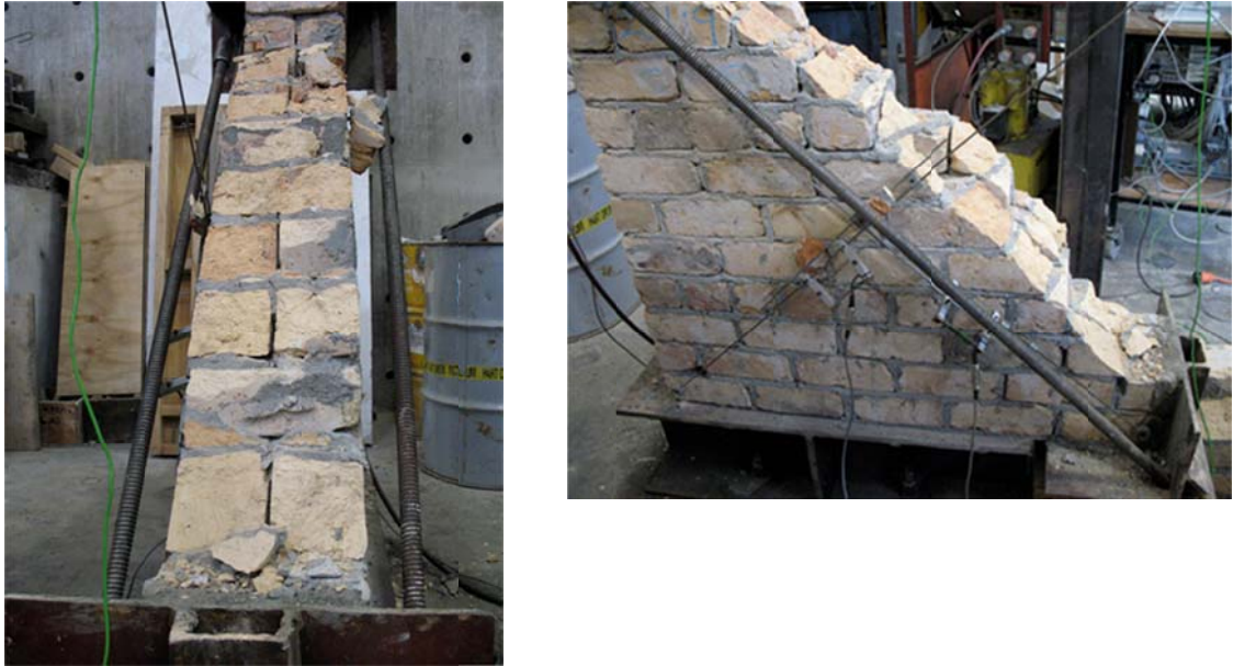
(b) Diagonal tension cracks to brick masonry. Note splitting of bricks, indicative of mortar stronger than bricks (Russell 2010)
