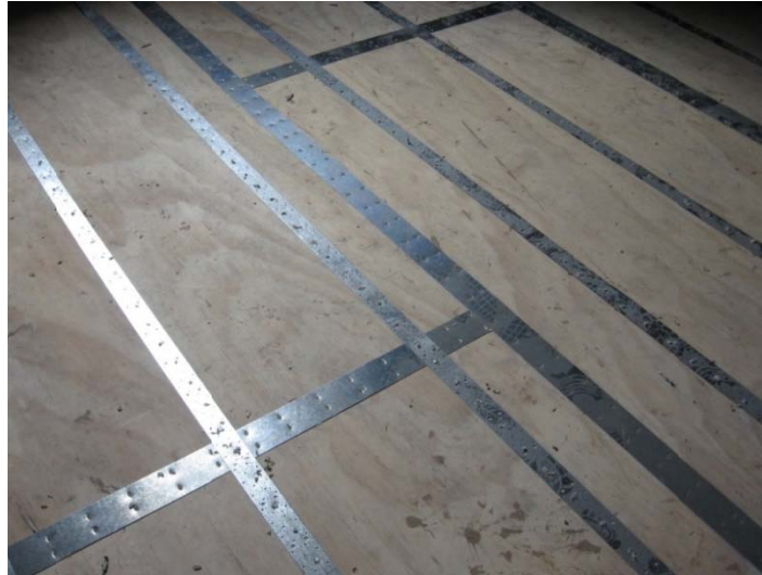
Figure 10.25: New plywood diaphragm (Holmes Consulting Group)
