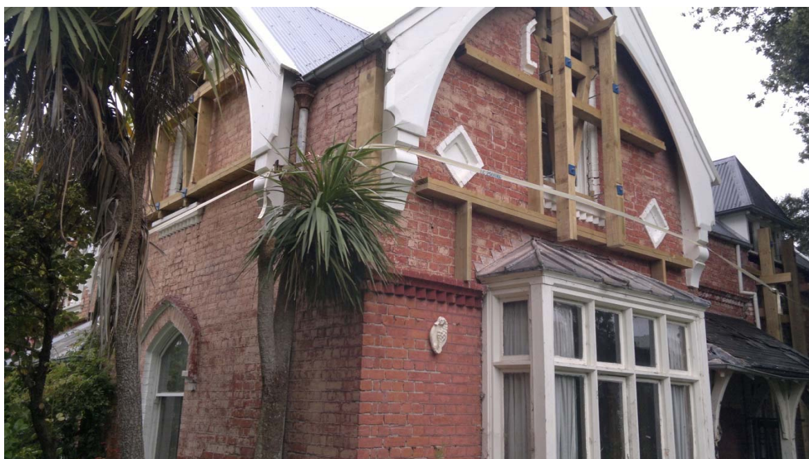
Figure 10.1: Temporary securing of a mildly damaged solid masonry URM building (Dunning Thornton/Heartwood Community)
