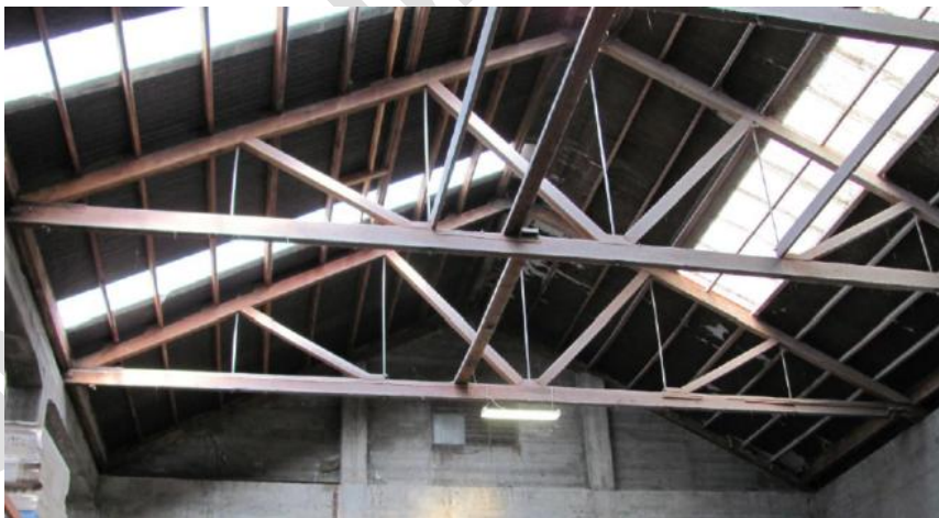
Figure C2E.1: Example of a flexible diaphragm
