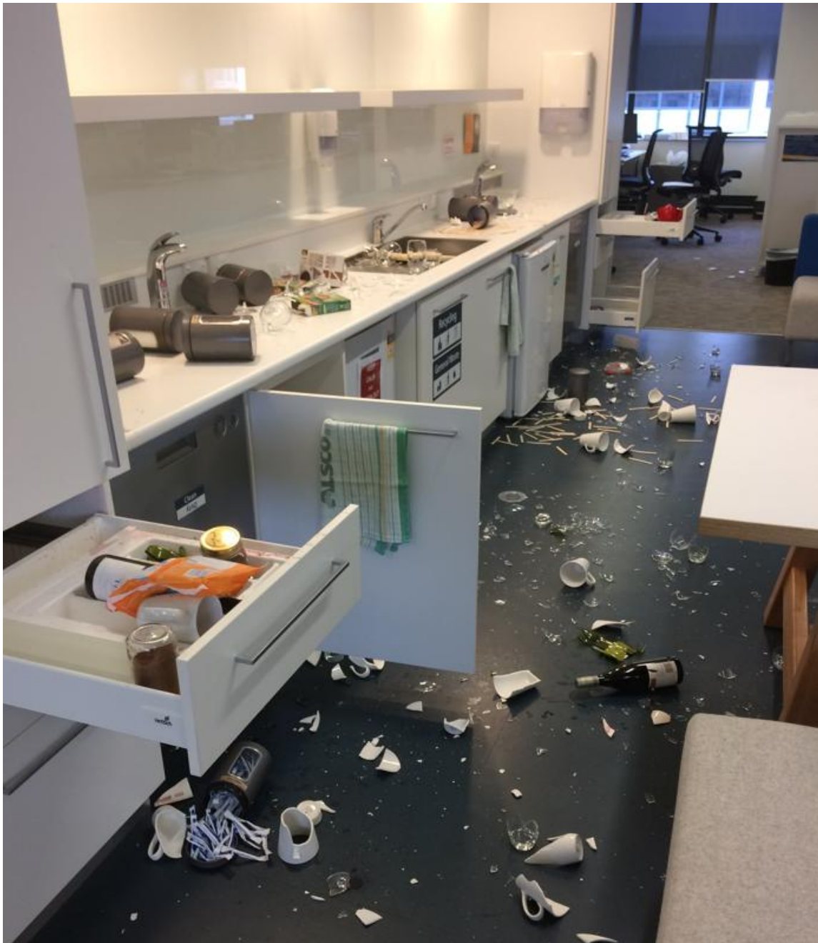
Figure 3-1: Example of building damage that could be expected at SLS1. Damage generally limited to building contents. Repairs to the building are not expected (Photo credit Beca Ltd, Damage from Kaikōura earthquake 2016).
