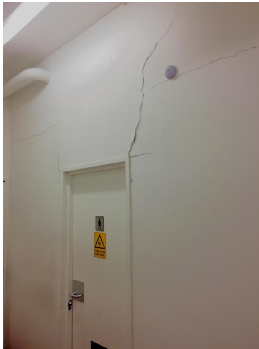
Figure 3-2: Example of building damage typical of DCLS where some damage is expected (cracking to non-loadbearing plasterboard partition walls shown). Extent of damage is expected to be limited to a level that is economically repairable (Photo credit Beca Ltd, Damage from Kaikōura earthquake 2016).
