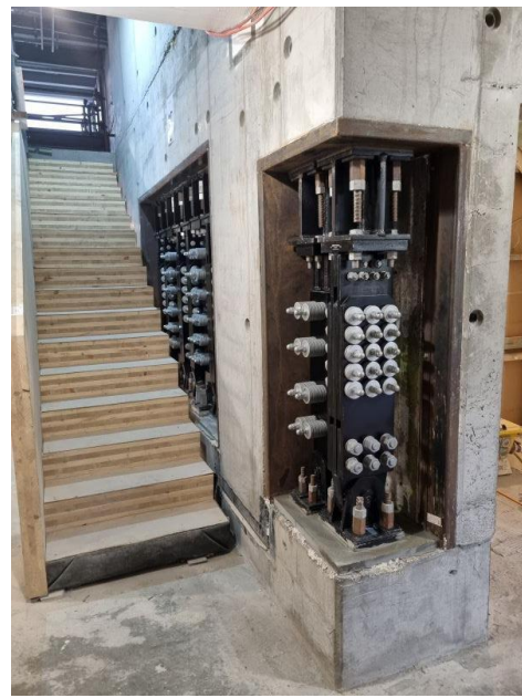
Figure D-12 Example of a friction damper systems (left) as a friction brace in a mass timber building (Fast + Epp, 2025) and (right) as a hold-down device in reinforced concrete structural wall (Tectonus, 2025)
