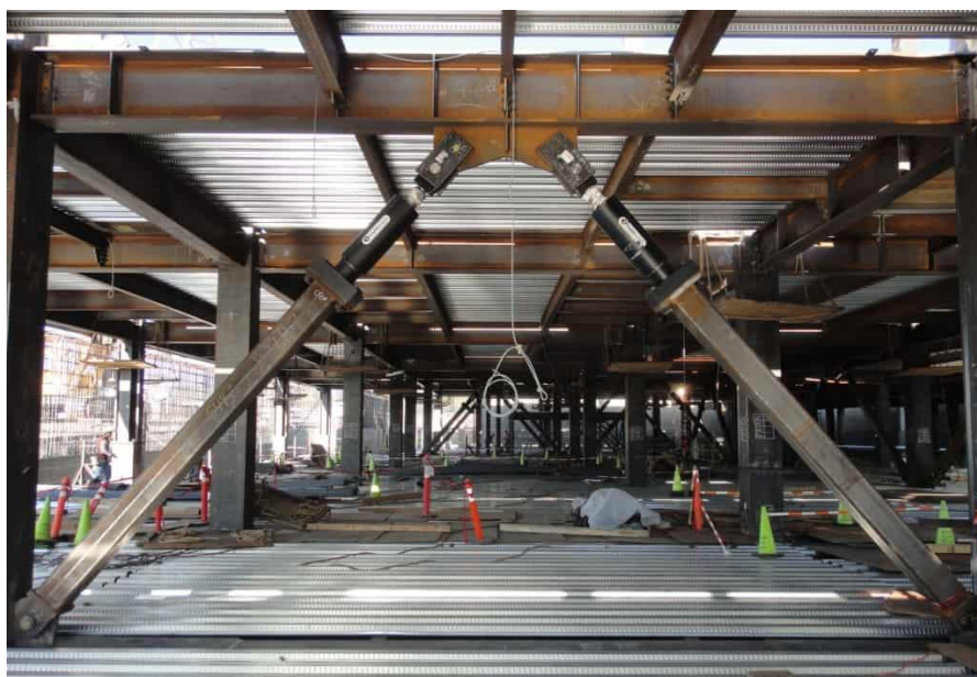
Figure D-11 Example of fluid viscous dampers in a steel structure (Taylor Devices, 2025).
