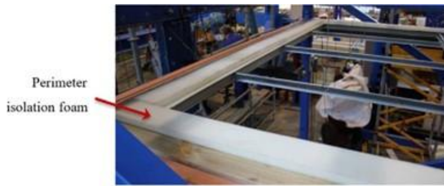
Figure 6-9 Isolation foam placed between ceiling framing and the timber boundary member (Pourali, Dhakal, MacRae, & Tasligedik, 2017).
